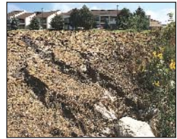
Soil erosion control
